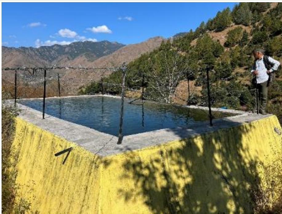
The storage tank at Saabli, built after the source catchment area was treated.
