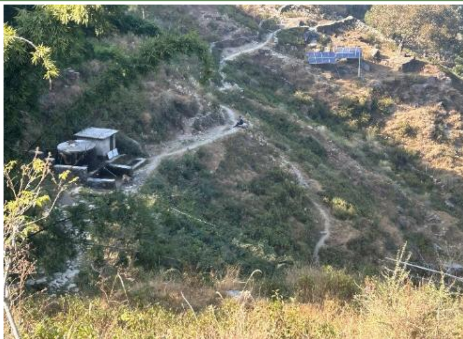
Solar panels and the collection tank installed above Monisakri village.
