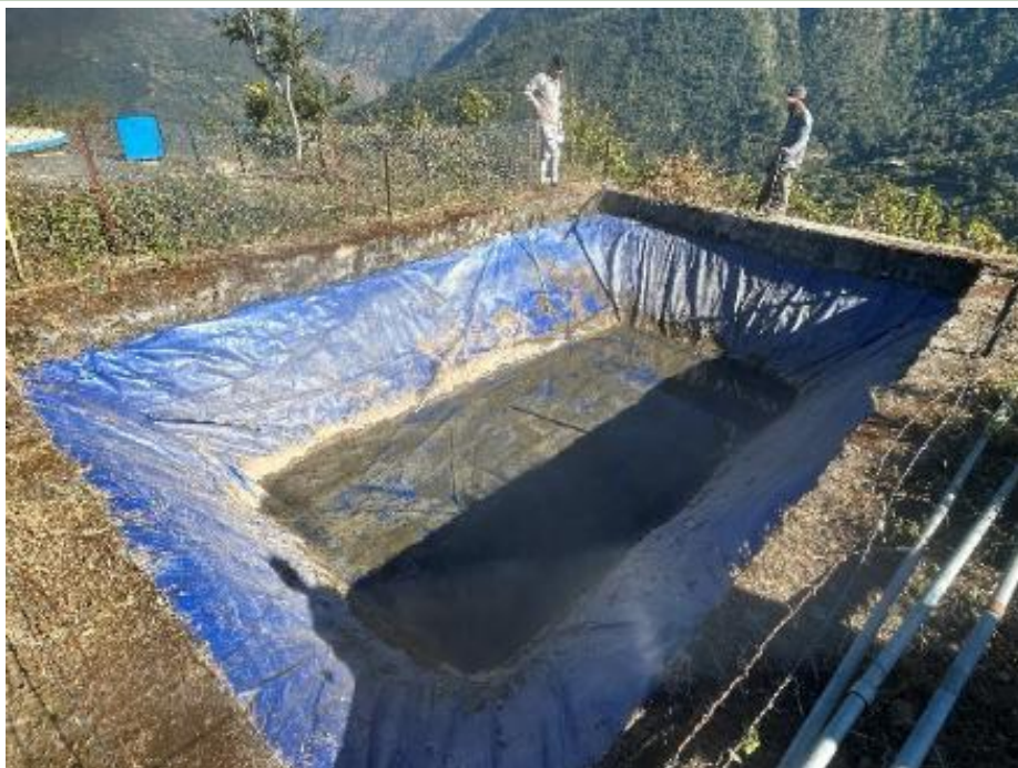
Construction of the LDPE storage tank at Taliya.
