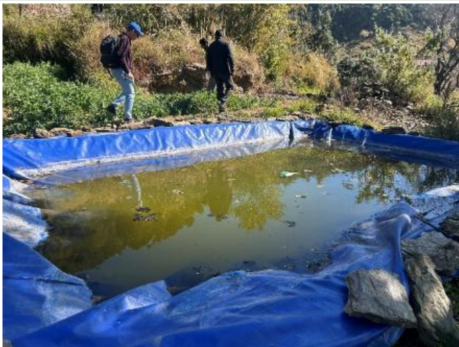
A rainwater storage tank at Chopriyalgaon.
