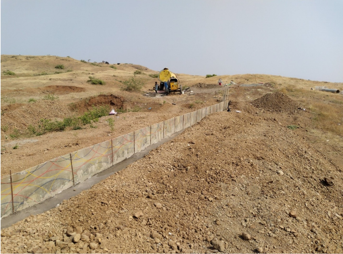
Figure 18. Fibre-sheet diaphragm being fixed midway along an earthen water-harvesting structure under construction at village Karjada, Bhavnagar district. (Photograph: Pidilite Industries / Triveni Kalyan Foundation.)
