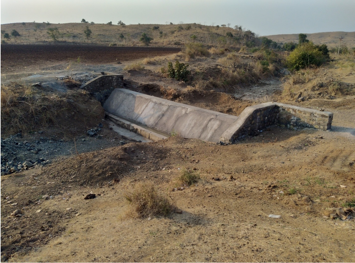
Figure 23. The completed composite hybrid check dam at village Karjada, with backfilling of soil still pending. (Photograph: Pidilite Industries / Triveni Kalyan Foundation.)
