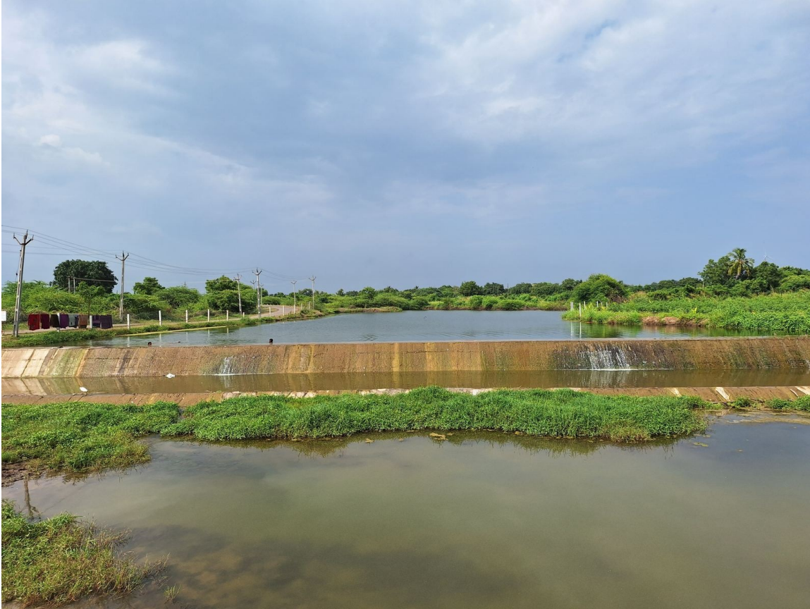
Figure 26. A percolation tank overflowing after the monsoon: water is held back by a low concrete wall so it can soak into the ground rather than run straight off the catchment. (Illustrative photograph.)
