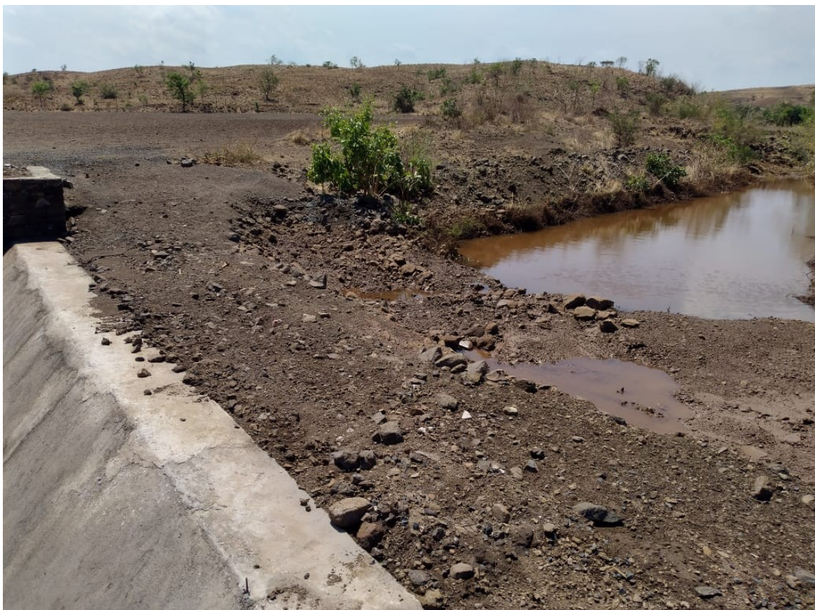
Figure 24. The completed hybrid check dam after its first monsoon flow, with the upstream pathway later added for carts, tractors and other vehicles. (Photograph: Pidilite Industries / Triveni Kalyan Foundation.)
