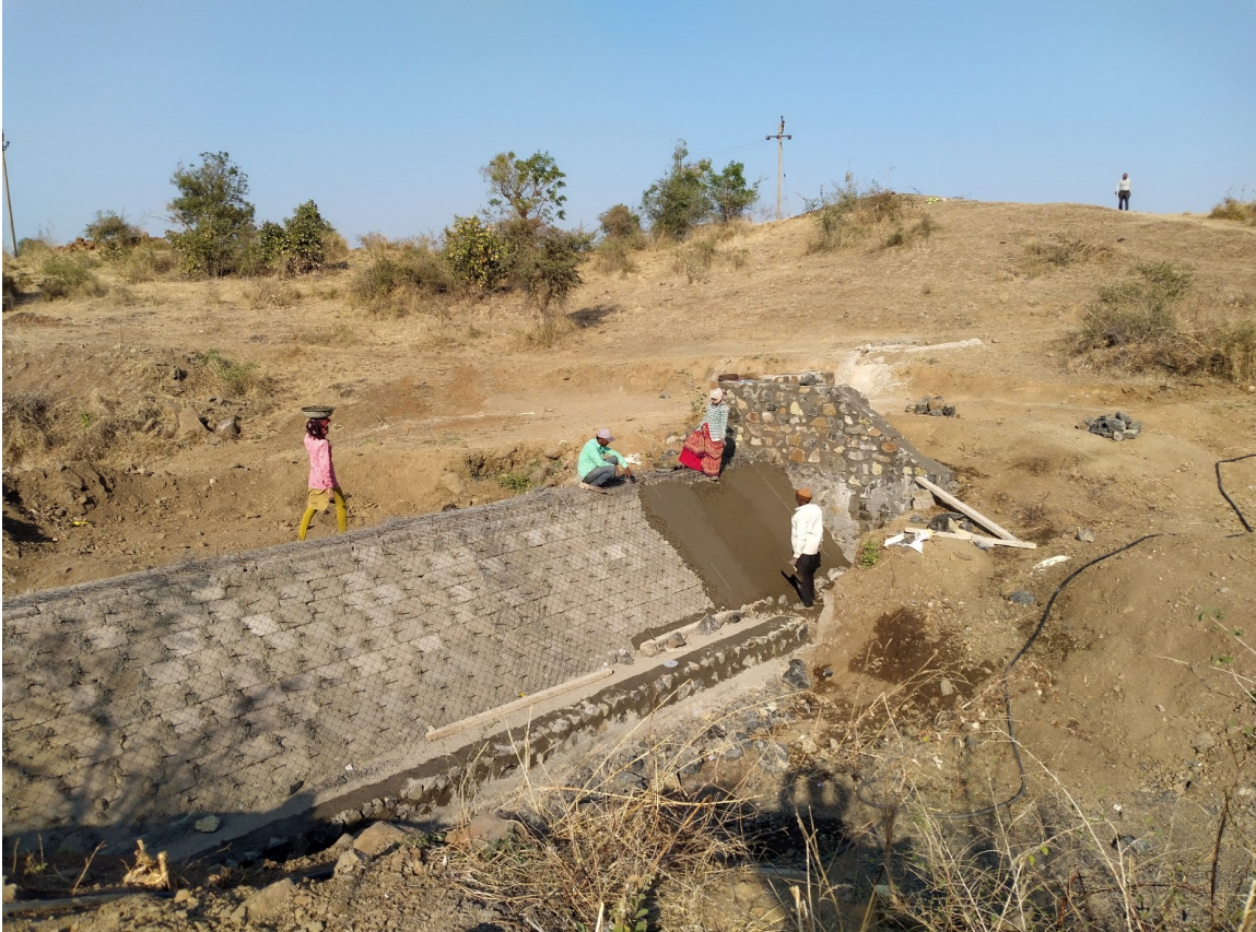
Figure 22. The low-cost composite hybrid check dam under construction at village Karjada, with its loose-boulder body wall, fibre-sheet diaphragm, earthen upstream support and GI-wire-mesh wrapping. (Photograph: Pidilite Industries / Triveni Kalyan Foundation.)
