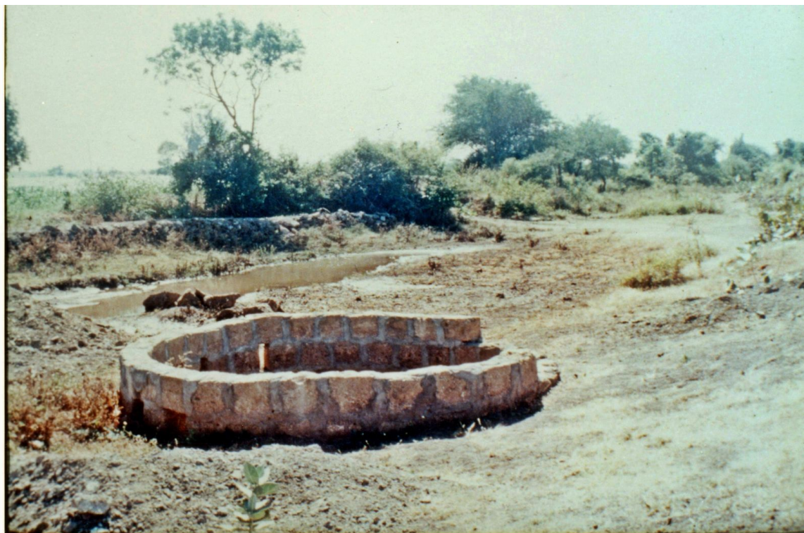
Figure 15. A circular masonry well-recharge structure, newly built and not yet in use, beside the channel that will feed it filtered monsoon runoff. (Illustrative photograph.)
