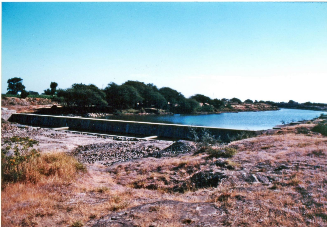
Figure 10. A completed weir holding back a broad stretch of impounded water on upwards side of its wall. (Illustrative photograph.)
