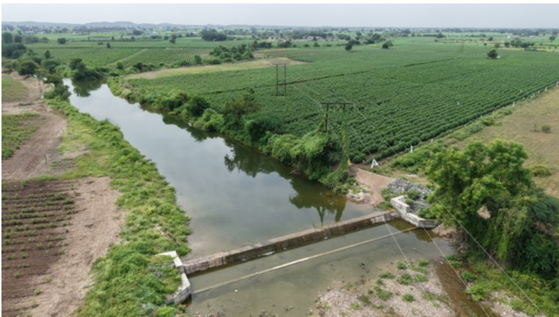
Figure 16. Check dam constructed at Sanosara, Sihor taluka, one of many structures built under the Pidilite programme across Bhavnagar district. (Photograph: Pidilite Industries / Triveni Kalyan Foundation.)
