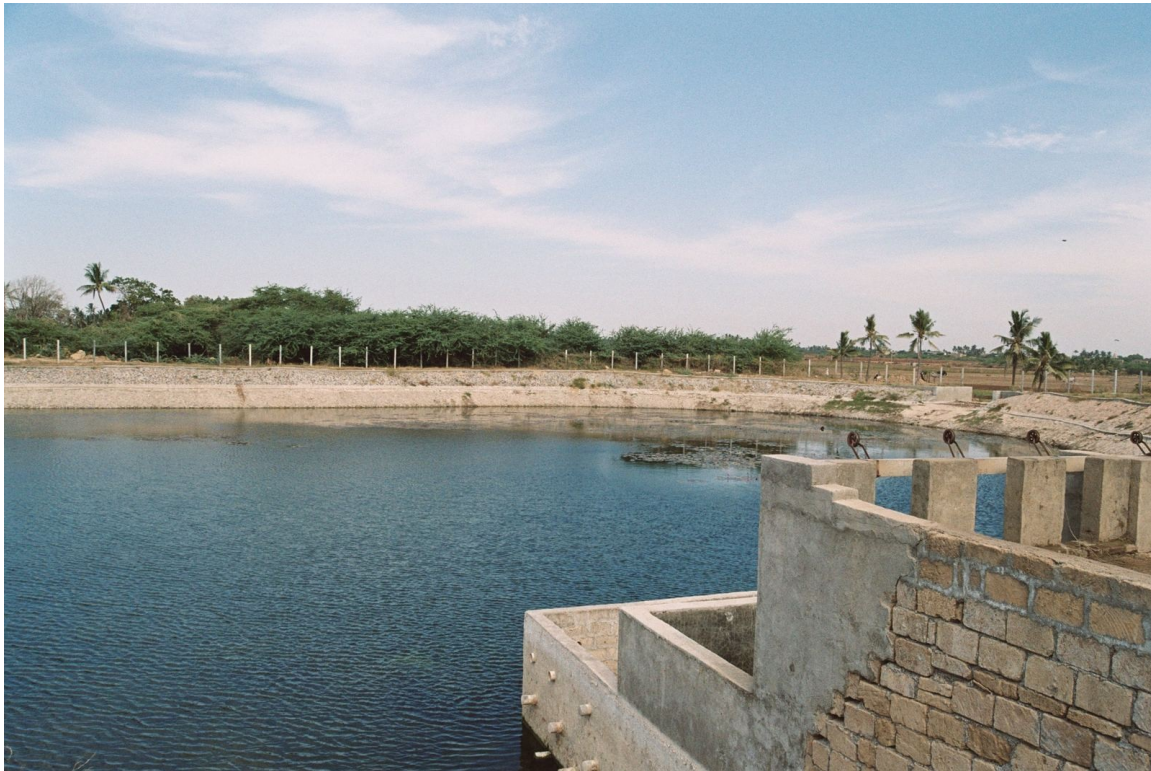
Figure 28. An open well-being recharged by the storage area of a percolation tank. (Illustrative photograph.)
