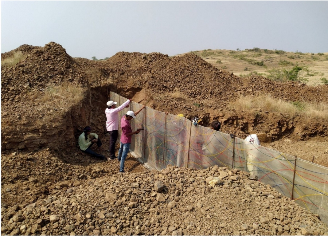
Figure 19. Fibre-sheet fixing under progress on the same earthen structure at village Karjada. (Photograph: Pidilite Industries / Triveni Kalyan Foundation.)
