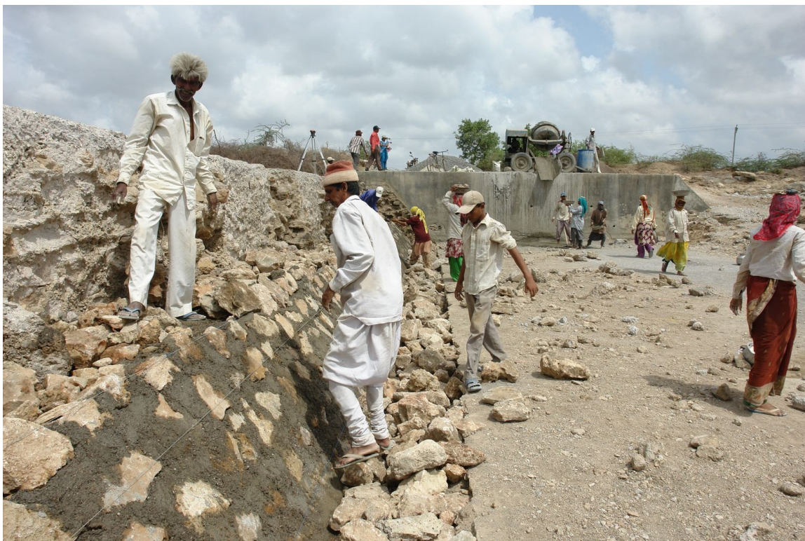
Figure 13. Villagers and masons build up a rubble-and-mortar check dam wall by hand — the kind of direct, supervised labour contribution that gave communities a stake in construction quality. (Illustrative photograph.)
