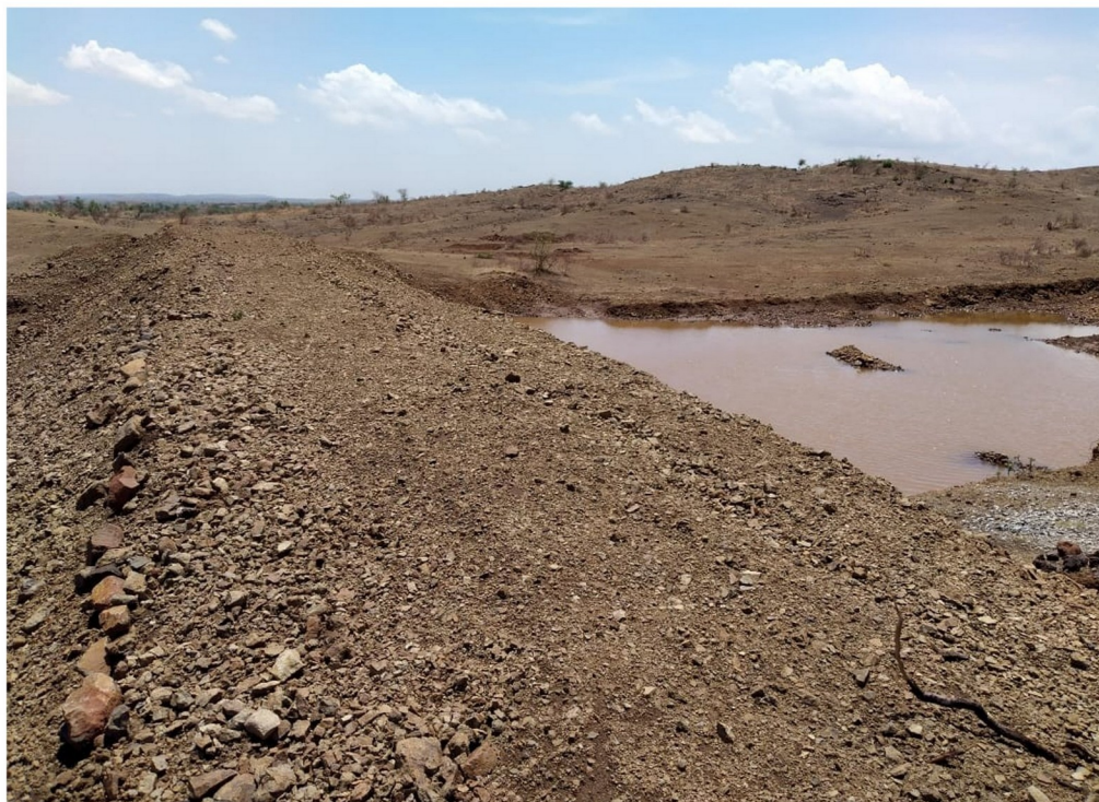
Figure 20. The same earthen water-harvesting structure holding water for the first time after completion, using borrow material from the spread area and an end-located free-flow waste weir. (Photograph: Pidilite Industries / Triveni Kalyan Foundation.)
