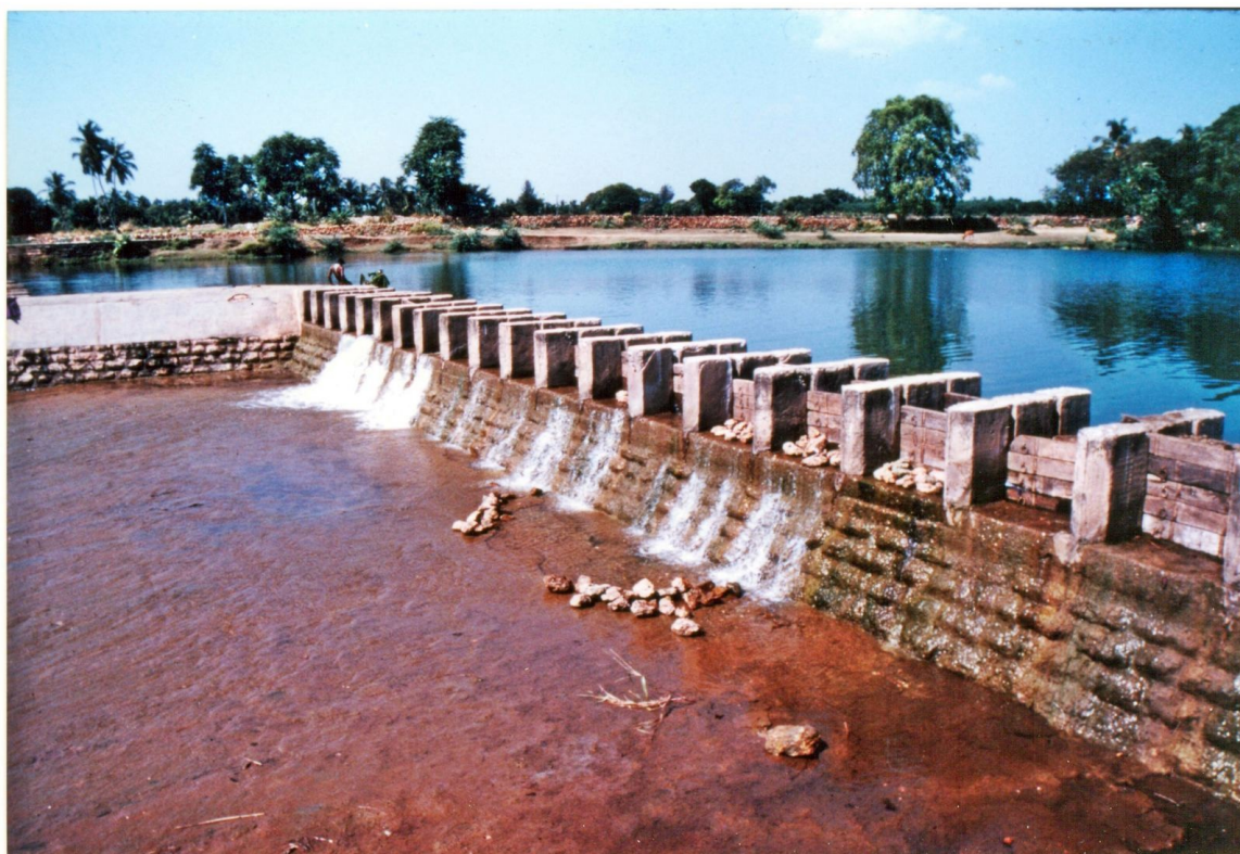
Figure 6. A completed check dam's stepped spillway in full flow, water cascading through each notch into the stream below — one of the movement's more substantial structures. (Illustrative photograph.)
