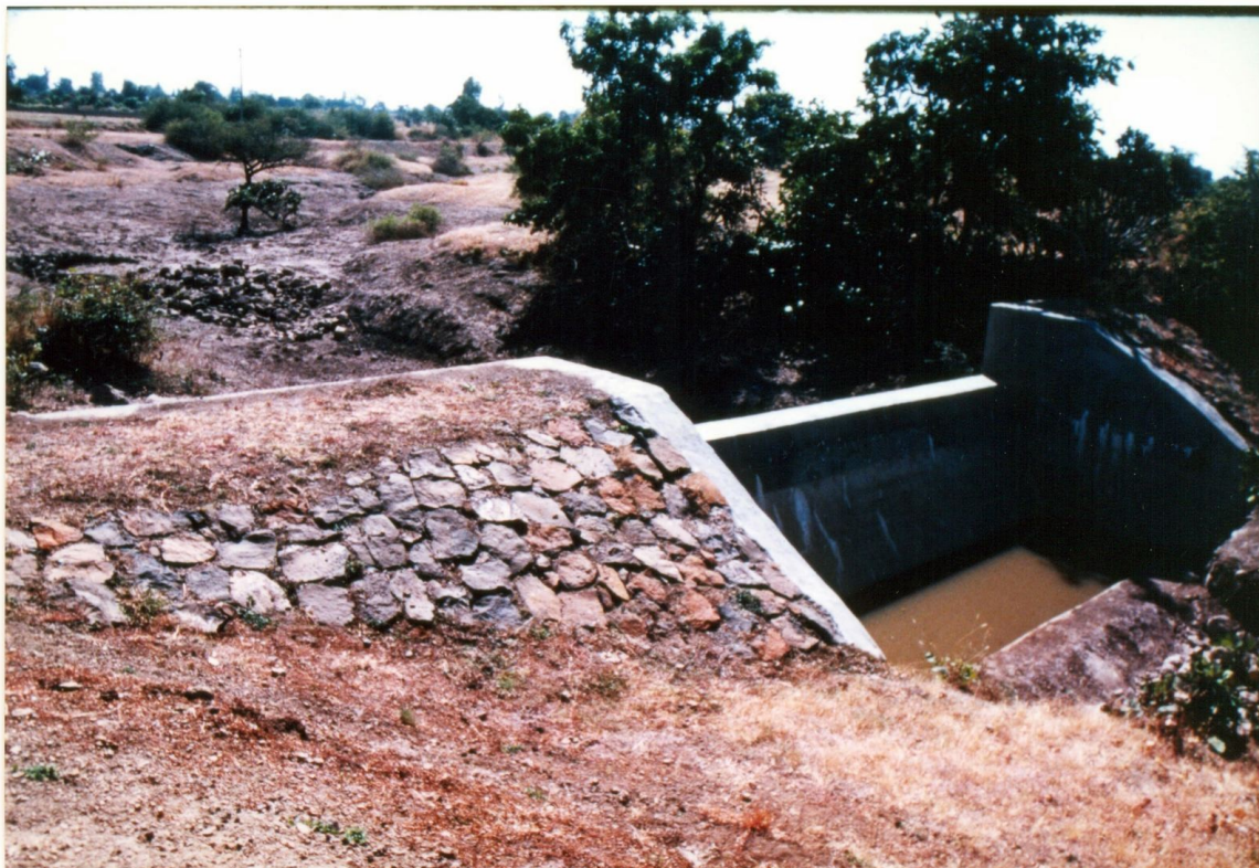
Figure 14. A small masonry outlet structure, water pooling behind it — the modest, locally built infrastructure typical of community-financed recharge works. (Illustrative photograph.)
