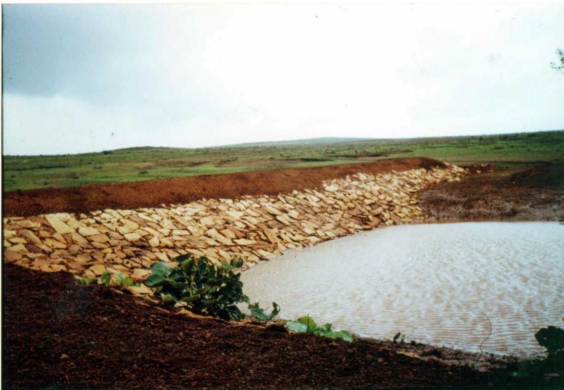
Figure 9. Dry rubble-stone pitching being laid along an embankment under construction, with water already backing up behind it — the kind of "hardware" that most NGOs of the period left to government contractors. (Illustrative photograph.)
