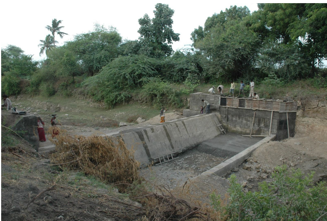
Figure 11. A check dam under construction on a Saurashtra streambed: villagers and masons work alongside the concrete shuttering and mixer, the kind of joint construction effort through which communities supervised quality and built a stake in the finished structure. (Illustrative photograph.)
