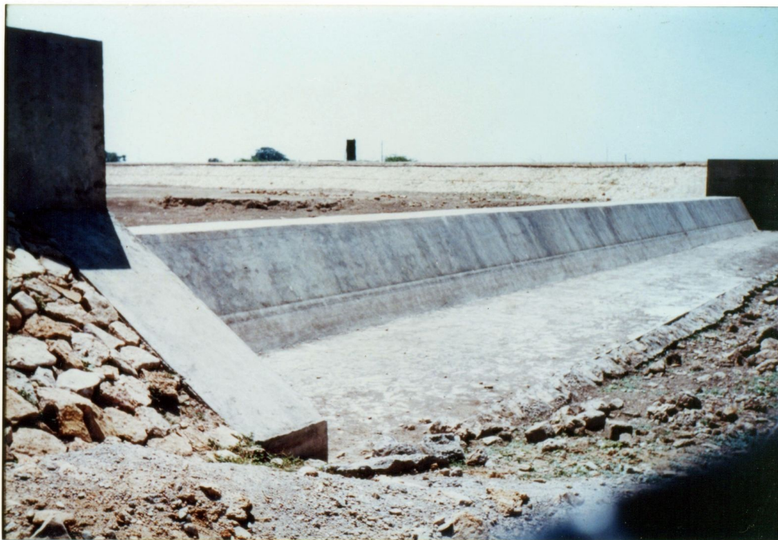
Figure 8. A check dam's spillway and wing wall photographed dry, well before or after the monsoon flow it is built to hold back — a reminder that a check dam's value lies mostly in water that has already soaked away, not in what is visibly standing. (Illustrative photograph.)
