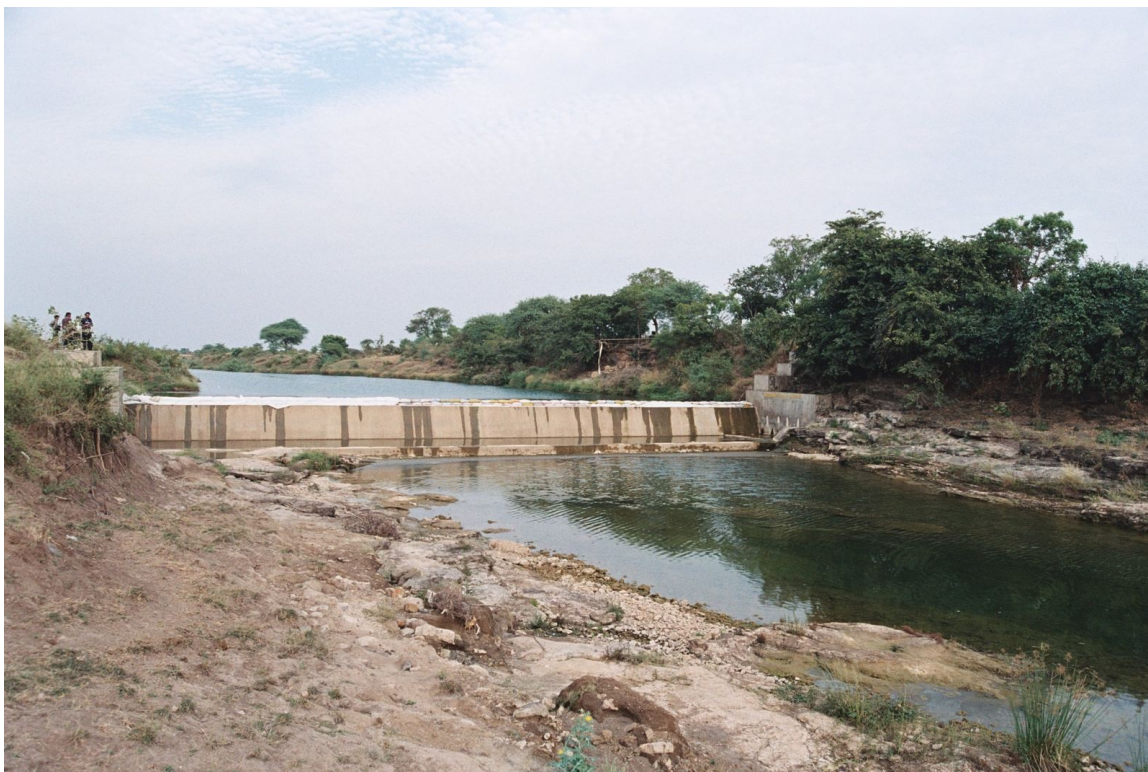
Figure 7. A masonry check dam across a Saurashtra streambed, holding back monsoon flow so it can infiltrate the aquifer beneath rather than run off to the sea. (Illustrative photograph.)
